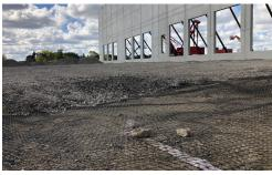
TriAx® Geogrid was used for this warehouse distribution site for its high performance and ability to extend maintenance cycles.
