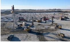
640,000 Sq. Ft. Fulfillment Center: Bondurant, Iowa 7,600 Geopier® elements piers were constructed in 48 days, shaving three weeks from the construction schedule.
