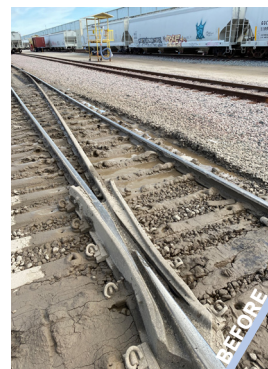
KTN Industrial Track Before Installation
