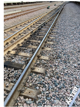
KTN Industrial Track After GeoSpike SM Installation
