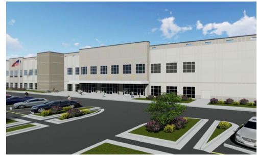
855,000 Sq. Ft. Distribution Center: Cleveland, Ohio Maximum column loads up to 710 kips, wall loads up to 10 klf. 6,400 Geopier® elements were constructed in six weeks.
