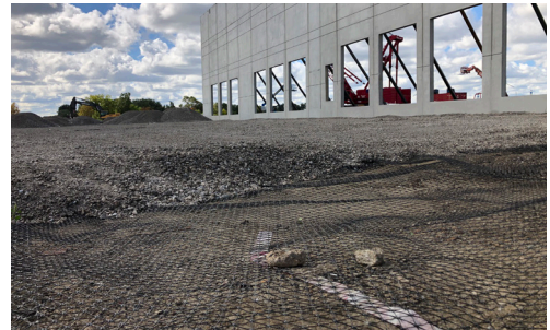
TriAx® Geogrid was used for this warehouse distribution site for its high performance and ability to extend maintenance cycles.
