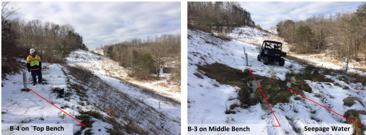
Figure 5. Inclinometer Locations and Its Surrounding Slope Conditions
