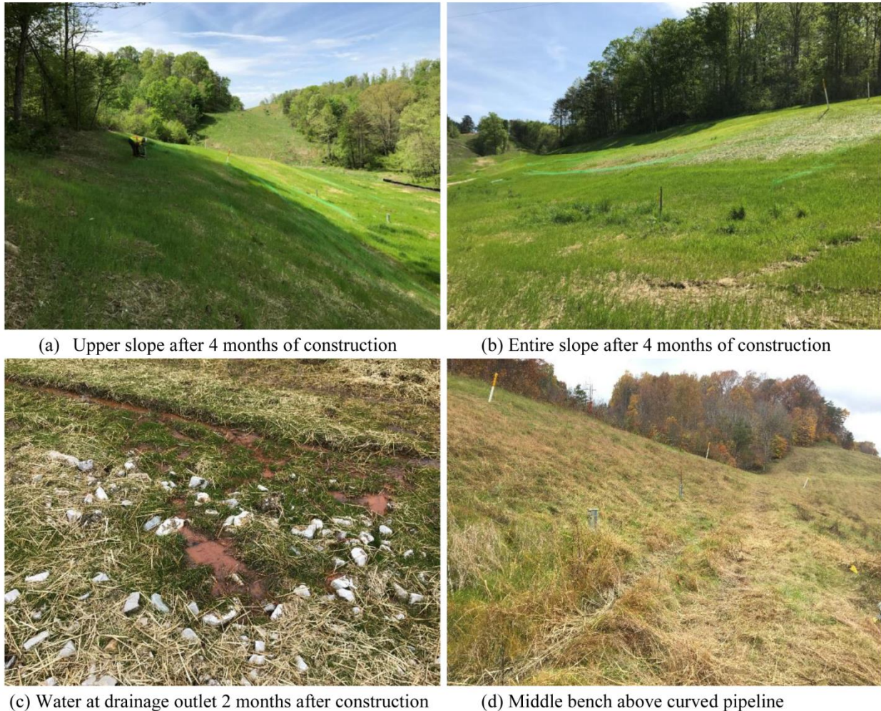
Figure 11. Inclinometer Locations and Its Surrounding Slope Conditions
