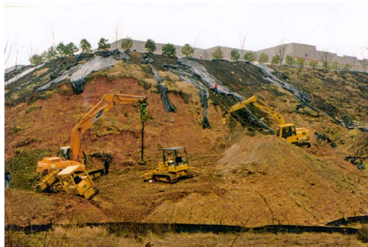
Figure 5: North Carolina landslide repair: during construction
