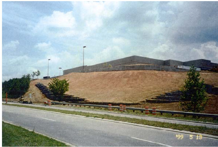
Figure 6: North Carolina landslide repair: after construction
